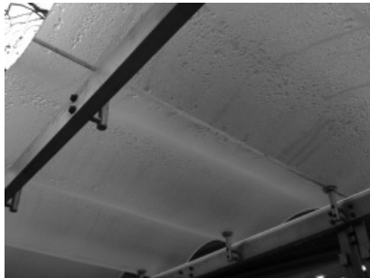
Seam connecting roof sections.
